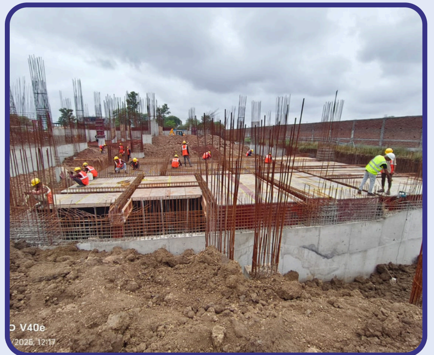
On Going Project Mandana 5 Star Hotel (Ujjain M.P.)
